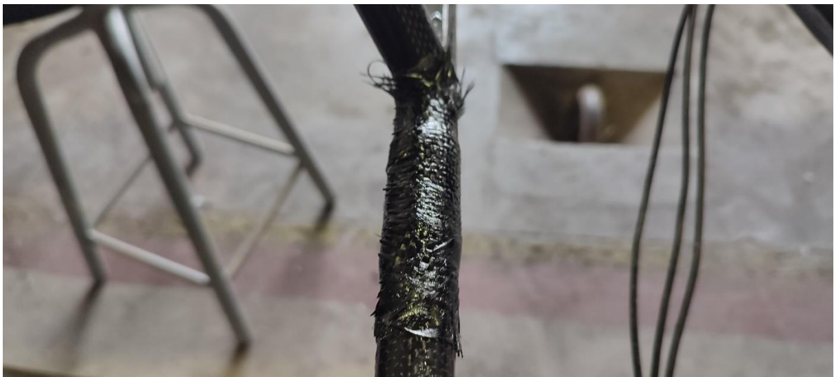
Figure 96 CF tape adjacent to a "T" joint in the boom
