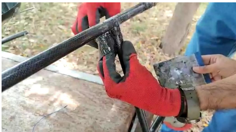
Figure 98 Using scraper to wind the tape tightly
