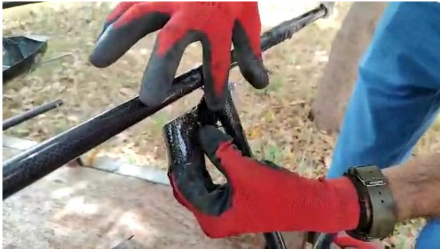
Figure 97 Taping up the T-joints
